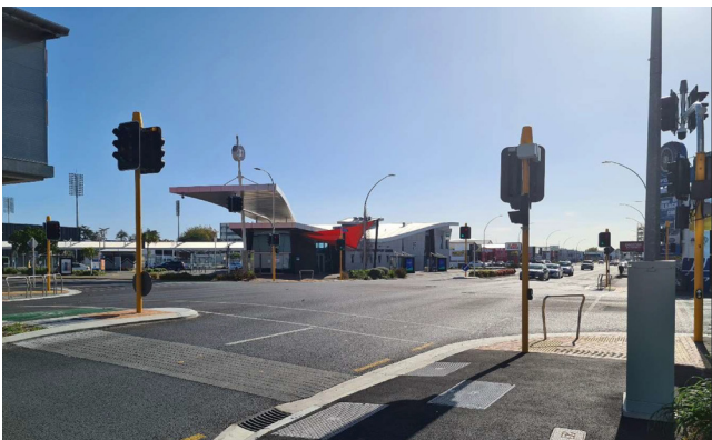
Trafinz Road Safety Leadership Award Hamilton City Council: 'Raised Safety Platform and Upgrade to Signalised Intersection: Anglesea Street/Bryce Street, Hamilton'
